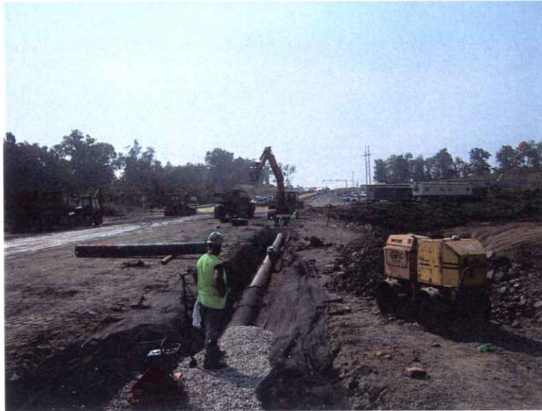
Installing Combination Storm Sewer.
