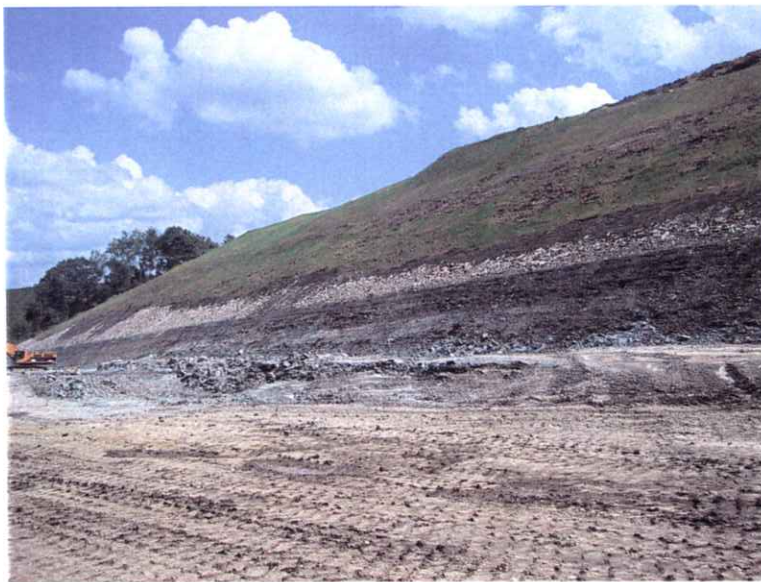
Slopes With Coal Seam Treatment Visible
