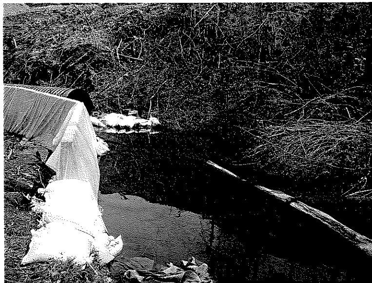
Stream Diversion In Jennings Run
