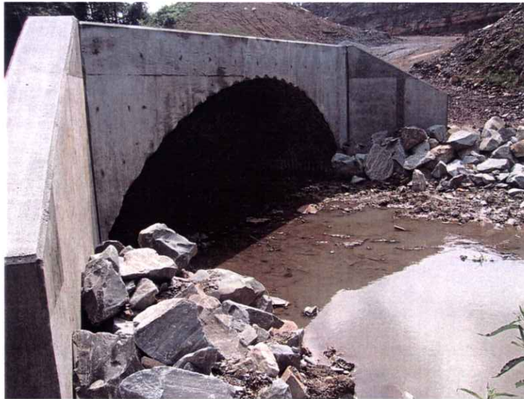
S-26693 with complete end wall, wing walls and scour protection.
