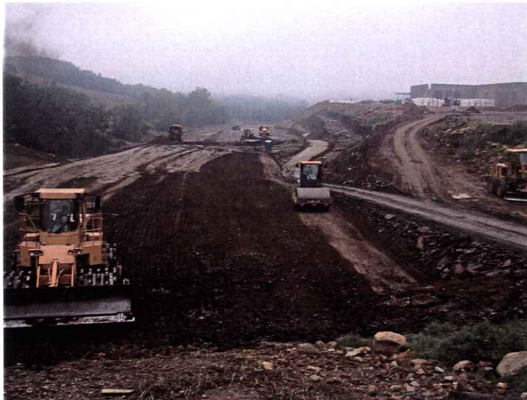
Embankment Placement
