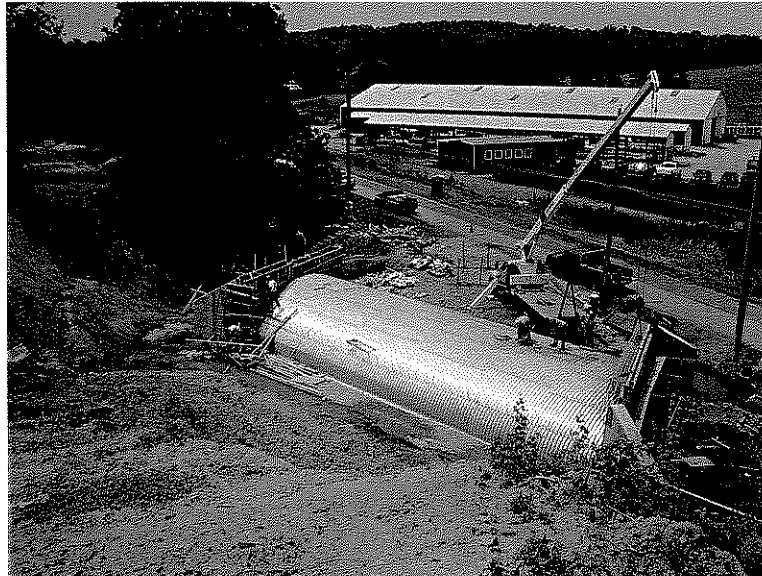
Complete Steel Plate Arch with Rebar and Forms for End Walls
