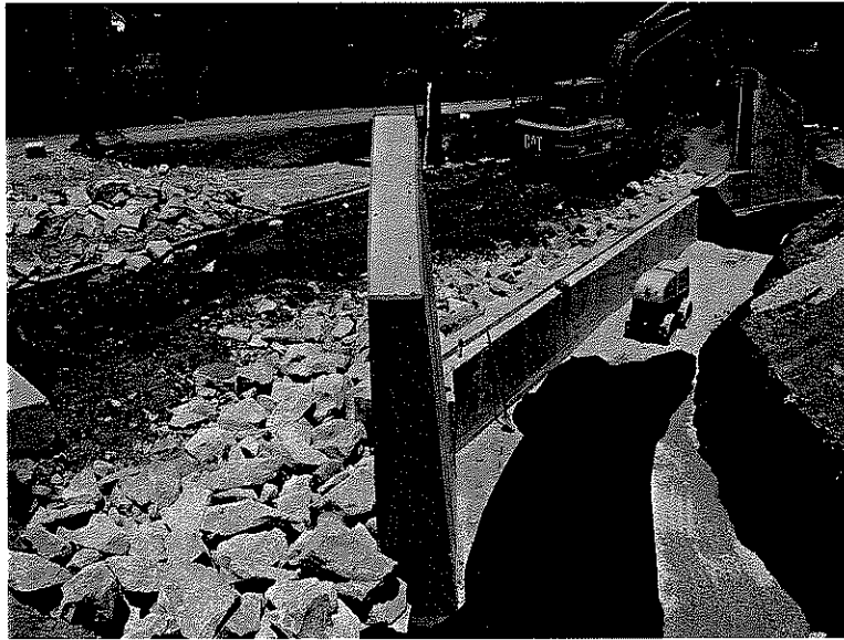
Limestone Structure Backfill and Scour protection along the South Foundation
